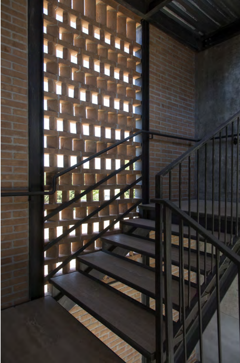
Figure 16. Brick “transenna” structures, closing and not load-bearing, in the stair towers.
