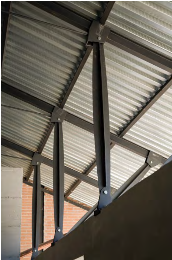
Figure 9. Detail of the struts supporting the roof steel structures.
