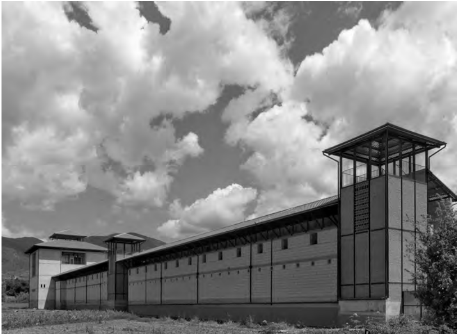
Figure 13. The continuous external wall facing the countryside.
