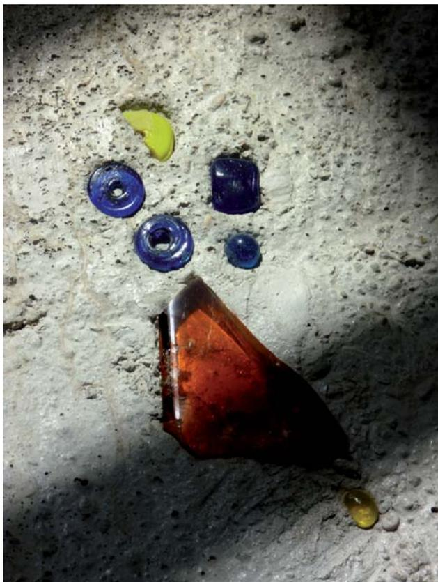
**Figure 17.** Detail of the votive chapel wall behind the altar: Coloured glass set on the concrete, washed with a jet of water to make the aggregates emerge.
